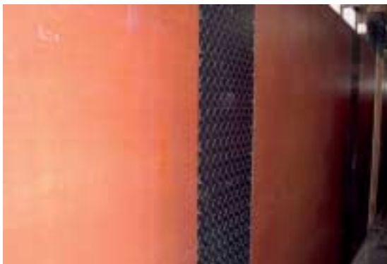
Fig. 8 The bridge slabs are manufactured in upright position; suitable metal sheets are attached to the form to obtain the roughness required for the glued joint.
