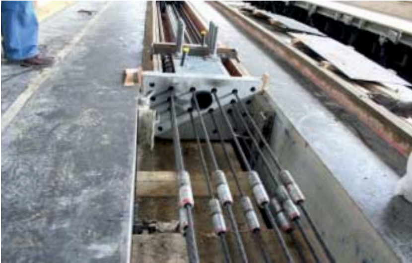
Fig. 7 The upper chords are prestressed with 10 strands. The corrugated sheath in the center of the slender girder is required for post-tensioning the individual elements after erection.
