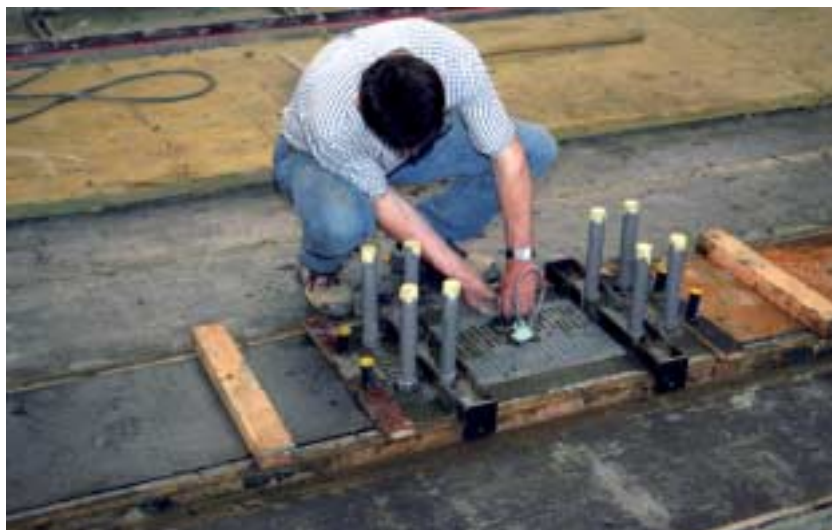
Fig. 10 Temperature sensors in the precast part for continuous checking of the hardening temperature.
