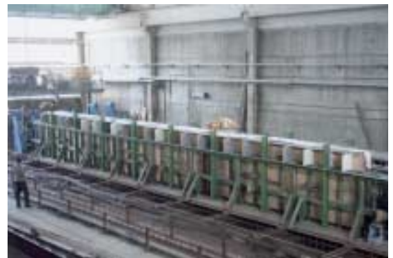
Fig. 8 The bridge slabs are manufactured in upright position; suitable metal sheets are attached to the form to obtain the roughness required for the glued joint.
